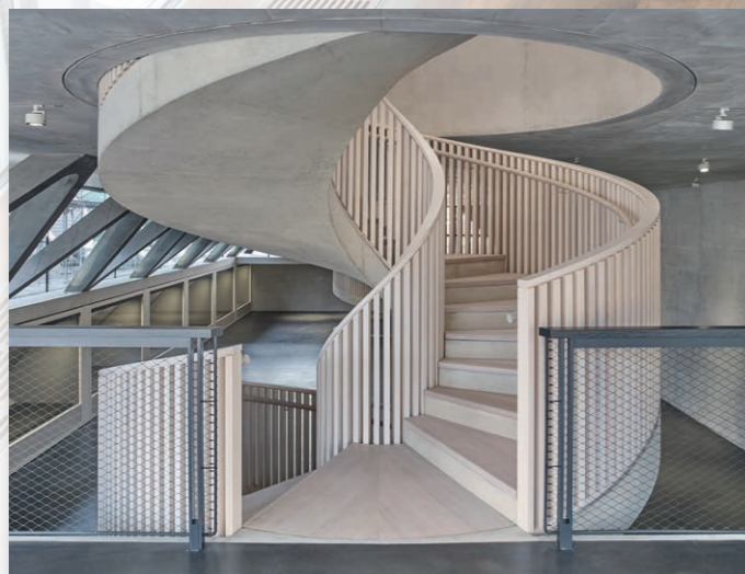
Spiral staircase at the centre of an administrative building of SSB. A filigree wooden staircase has been built around a load-carrying concrete structure.
